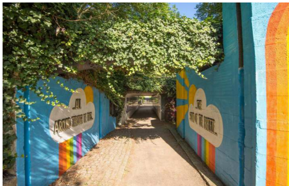
Figure 23 National Cycle Route 1 underpass below Lea Bridge Road
