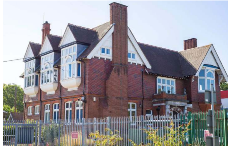
Figure 45 Thames Water Site - Engineer's House
