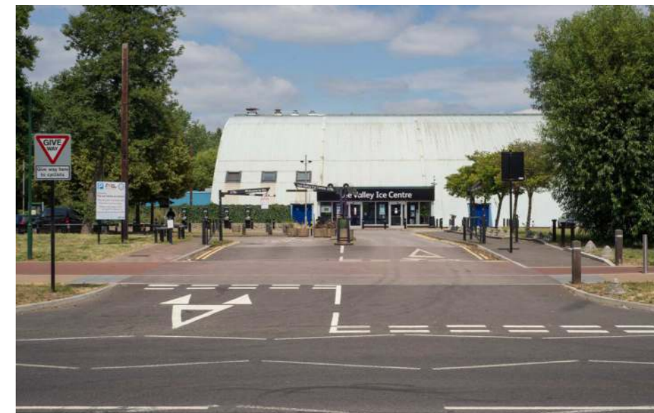
Figure 8 Existing LVIC access from Lea Bridge Road
