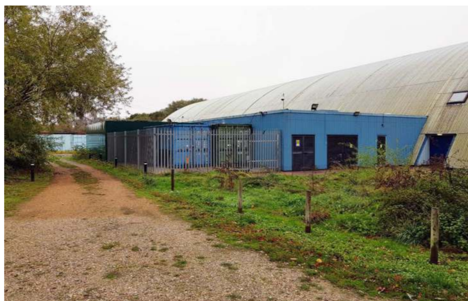
Figure 9 Existing LVIC plant area looking east from Sandy Lane
