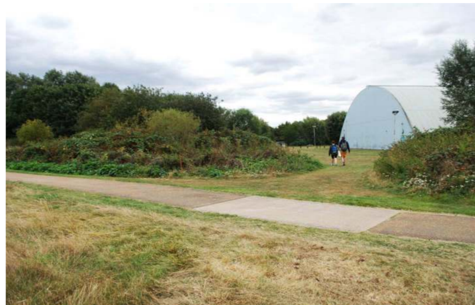
Figure 12 Existing LVIC from Greenway to north boundary of site
