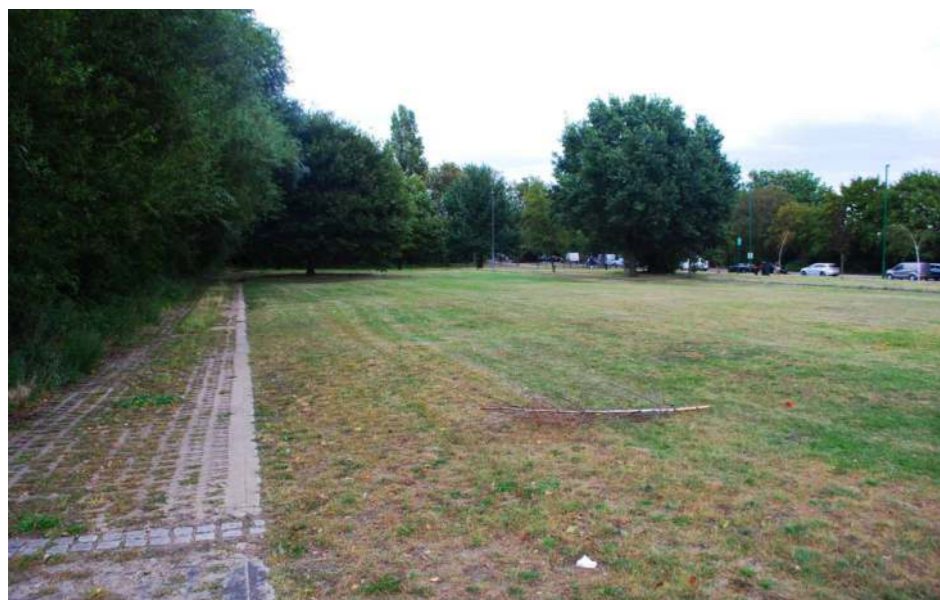
Figure 15 Existing grasscrete to Lea Bridge Road
