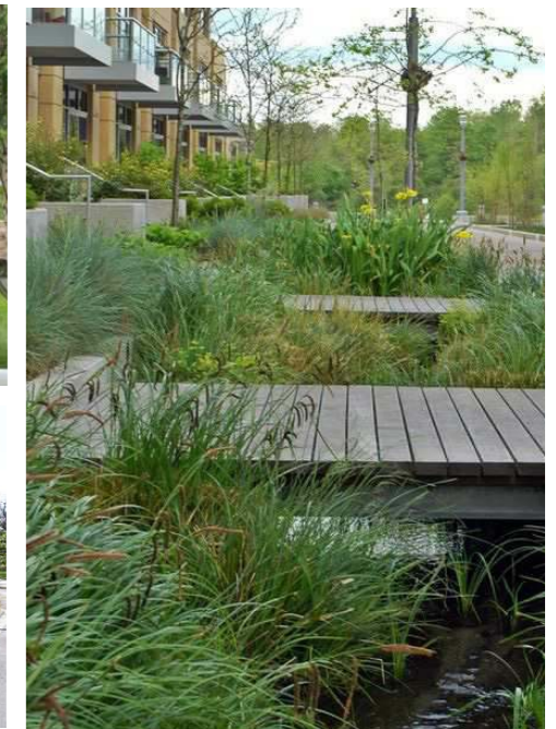
Timber swale footbridge
