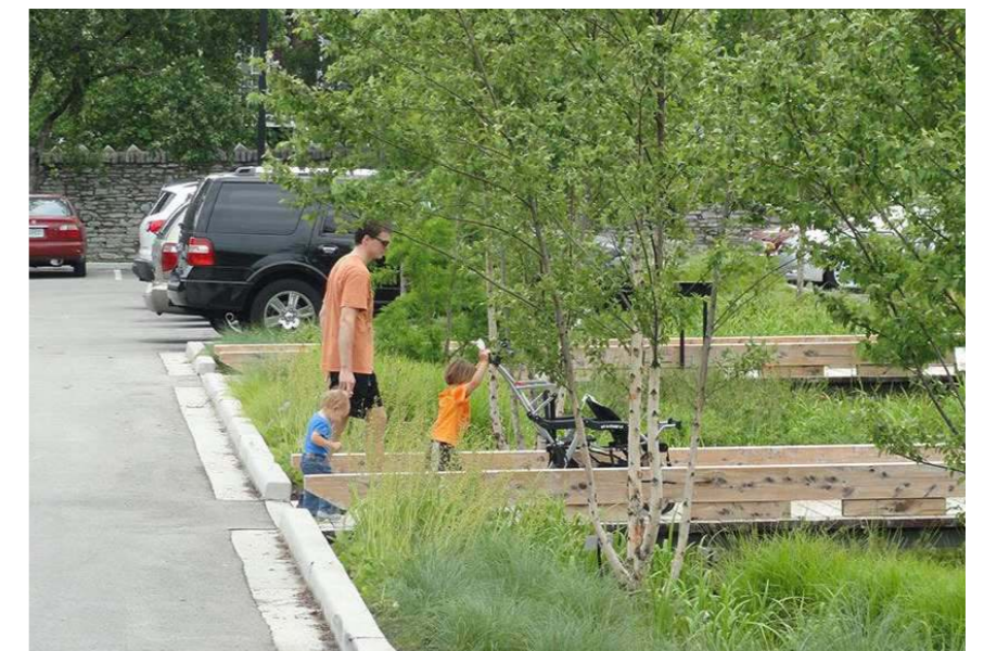
Figure 156 Bridges over swales
