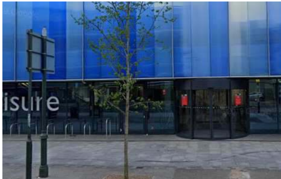
Figure 118 Similar entrance door installed at Sapphire Centre, Romford
